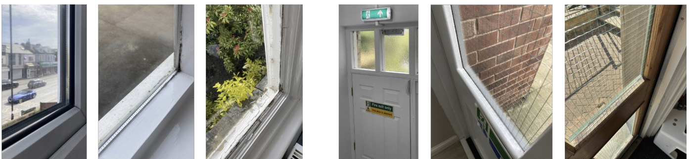
Left to right: newer double-glazed, old double-glazed, single-glazed windows, single-glazed fire doors.
