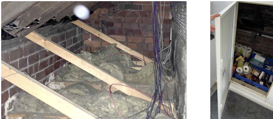
Scrambled loft insulation and uninsulated hatch
