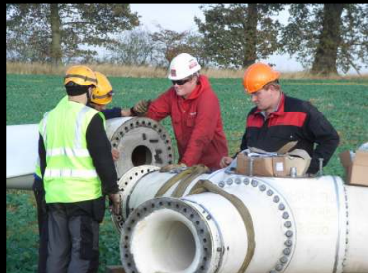
Assembling the rotor
